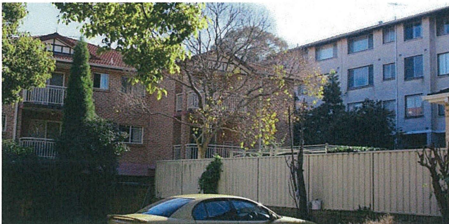
Figure 12: Residential Flat Buildings off Croydon Ave.
